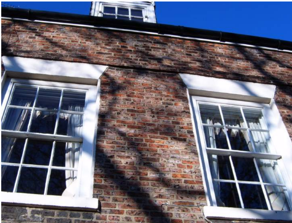
EXAMPLES OF THE EXISTING TIMBER SASH WINDOWS
